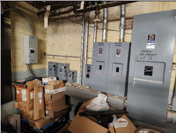
Front of building basement level
