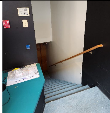
Basement stairs at front of building
