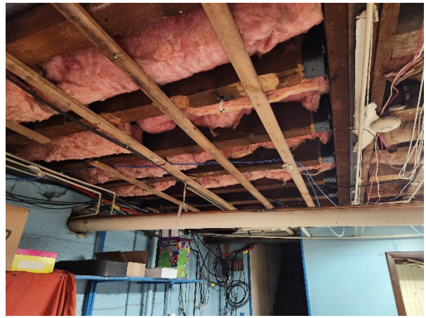
Example of ceiling in basement area
