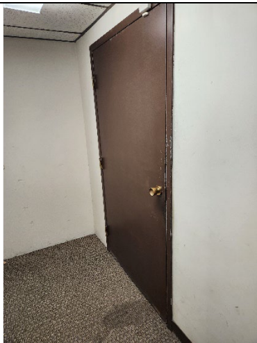
Entrance to basement area
