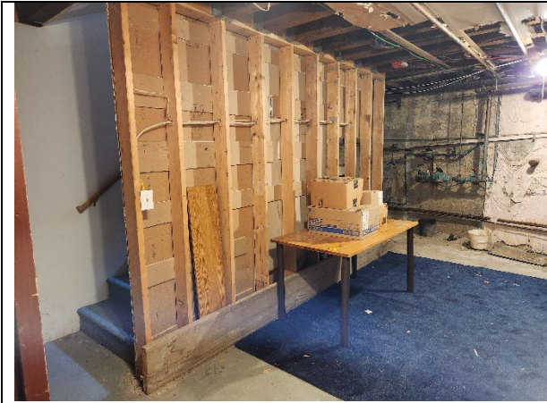
Basement stairs exiting to front of building.
