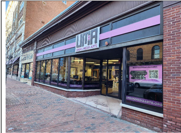
Front of building
