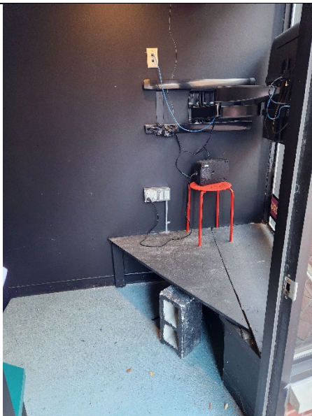
Basement entrance at front of building
